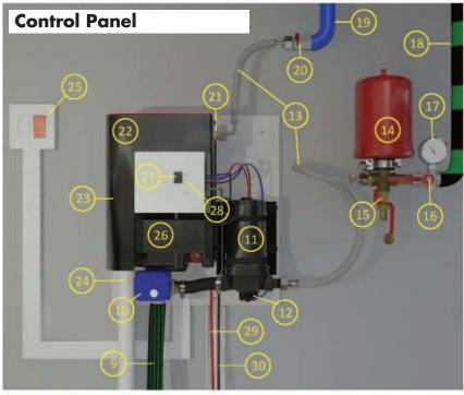
When in operation both valve 16 and 20 must be in the open position.
