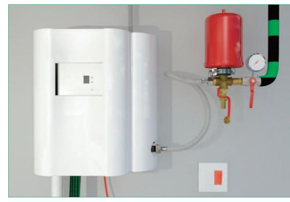
The StormSaver control panel is the central hub of the system. All the rainwater must pass through here on its way to the points of use. The control panel is the place where all the different pipes and hoses connect up, and should be considered when choosing its location within the building. The unit comprises of the pump, a small water storage tank, a pressure vessel and the electrical control panel which enables the whole system to function and includes the display panel.
