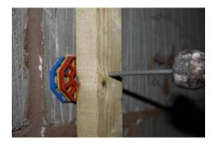
When filling a space or gap, always use the largest size possible to minimize the number of packers needed. The sizes of packers offered will, when used in combination, fill any gap in 1mm increments from 1mm upwards.
