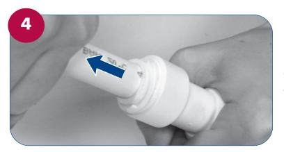
Check that the assembly is secure by pulling away the pipe from the fitting.
