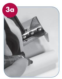
We recommend that you mark the insertion depth onto the pipe.
