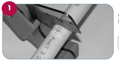
Cut pipe to size using pipe cutters (do not use a hacksaw).
