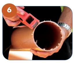
✓ Ensure all cut lengths of pipe are chamfered to roughly a 45° angle.
