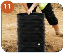
To complete the installation of Inspection Chambers, add risers to the required depth.
