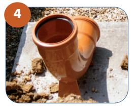
If fitting to a vertical soil and ventilation pipe, it is important to place a solid support under the long radius rest bend.
