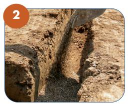
To ensure the pipe is supported correctly, drop in pea shingle to form the pipe bed.
