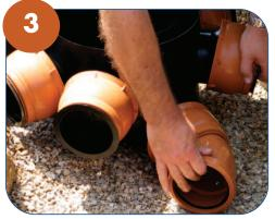
Plan out where the major fittings will sit. Ensure the inspection chamber is aligned so that the flow of water is maintained through the main channel to minimise any potential blockages.
