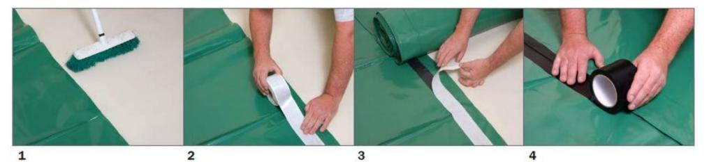
Ensure that the area is free from stones and mortar droppings as these could damage the membrane Roll out the first membrane and apply the Double Sided Jointing Tape 50mm in from the edge Position the second membrane overlapping the first by 150mm. Remove the backing paper from the Double Sided jointing tape approximately 1m at a time and unroll the second membrane. Pressure should be applied to ensure a good seal.
