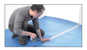
Butt the next row edge tightly to the first, ensuring that they do not overlap. Carefully tape the joints using a waterproof tape. All rows, including the last, should also be laid with a minimum of 20mm up the wall. This will be concealed behind the new or refitted skirting, scotia/trim once the floor is laid.
