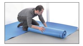
Ensure floor is clean and flat\*. Unroll at 90° to the direction of the floor, covering area to be laid. To assist laying, apply double-sided tape to the perimeter of the sub-floor.
