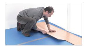
Lay the flooring on top of the **ACOUSTALAY®**, referring to the manufacturer's instructions.
