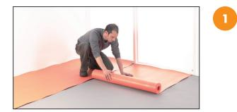
Ensure floor is clean and flat\*. Unroll at 90° to the direction of the floor, covering area to be laid. To assist laying, apply double-sided tape to the perimeter of the sub-floor.
