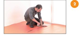
Butt the next row edge tightly to the first, ensuring that they do not overlap. Carefully tape the joints using a waterproof tape. All rows, including the last, should also be laid with a minimum of 20mm up the wall. This will be concealed behind the new or refitted skirting, scotia/trim once the floor is laid.
