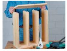
Then slide the Dowelmaster with the guide groove over the dowel, and drill. After this, apply glue to the boards.
