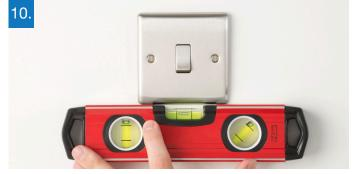
Insert and tighten the retaining screws provided. Use a spirit level to make sure that the socket is level. Restore the power at the consumer unit and test.
