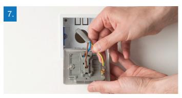
Place the brown wire (live) into the COM terminal, the switched live wire (blue/brown stripe) into the L1 terminal and the green/yellow wire (earth) into the separate earth terminal on the face plate.
