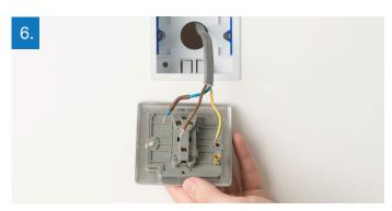
Line up the new switch and take note of where each terminal is located.
