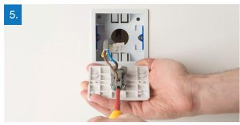
Unscrew each terminal to release the wires. You should now be able to remove the switch and place it to once side.
