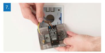
Place the brown wire (live) into the COM terminal, the switched live wire (blue/brown stripe) into the L1 terminal and the green/yellow wire (earth) into the separate earth terminal on the face plate.
