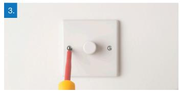
Test power is not supplied to the switch by using a plug in socket tester or multimeter. Unscrew the retaining screws on the switch so that it is released from the mounting box.
