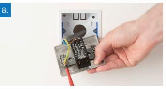
Make sure that the wires are fully inserted into the terminal and that no bare copper wire is visible. Tighten the screws securely onto the copper wire, not the outer sheathing.
