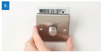
Gently press the switch back into place over the mounting box. Take care not to trap any wires between the wall and the switch.
