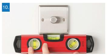
Insert and tighten the retaining screws provided. Use a spirit level to make sure that the switch is level. Restore the power at the consumer unit and test.
