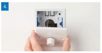
Gently ease the switch from the mounting box to show the wiring.
