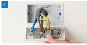
For this outlet there will be two sets of wires; one set for the supply (incoming power) and one for load (cooker).
