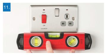
Screw the retaining screws provided. Use a spirit level to make sure that the socket is level. Restore the power at the consumer unit and test.
