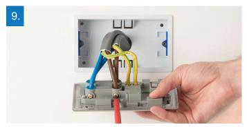
Make sure that the wires are fully inserted into the terminal and that no bare copper wire is visible. Tighten the screws securely onto the cable.
