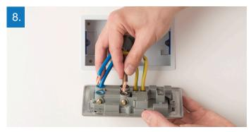
Noting supply and load, place a single blue wire into each neutral terminals, brown wires into the live terminals and the green/yellow wires into the earth terminals. There is one terminal for each wire.
