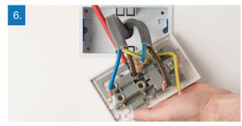
Unscrew each terminal to release the wires, noting supply and load. You should now be able to remove the socket and place it to one side.
