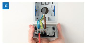
Make sure that the wires are fully inserted into the terminal and that no bare copper wire is visible. Tighten the screws securely onto the copper wire, not the outer sheathing.
