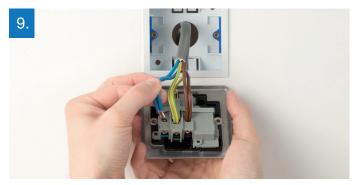
Place the blue wire(s) into the neutral terminal, brown wire(s) into the live terminal and the green/yellow wire(s) into the earth terminal. The terminals on the socket are colour-coded to help locate the correct one.
