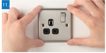
Gently press the socket back into place over the mounting box. Take care not to trap any wires between the wall and the socket.
