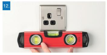
Insert and tighten the retaining screws provided.
