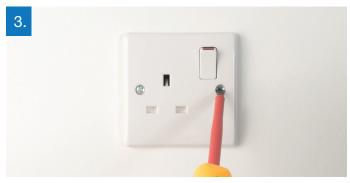
Test power is not supplied to the socket by using a plug in socket tester or multimeter. Unscrew the retaining screws on the socket so that it is released from the mounting box.
