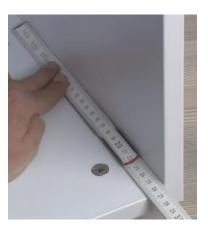
7. Selecting the runner marked DL and using the mark made in step 6, fit the runner to the inside of the cabinet so that the wheel is positioned as per the diagram below.
