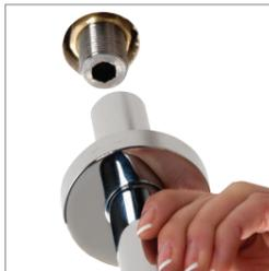
**5** Temporarily cap off the end of the shower arm and turn on the shower to pressurise the system and check for leaks. If all is sound, turn the shower off and remove the blanking cap (remembering the system may be under pressure).
