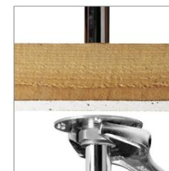
**7** Cut off the excess pipe allowing for a suitable working length to allow for the required 22mm connection. If a push fit connector is to be used then the pipe must be abraded to remove all chrome plating.
