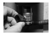
When using the key/cap to bleed air from the system make sure you have a bucket handy to catch the spill. Screw key/cap onto drain valve as a drip cover
