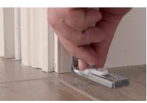
**5a.** Offer the door up to the opening to identify where to position the top pin pivot and top roller guide.
