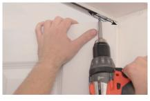
6. Unscrew and release the top pivot in the top metal track.
