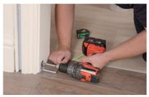
**c.** Slot the plastic pivot retainer into the bottom pivot bracket.
