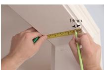
To determine which way to position the track, you will need to decide which way you want the door to fold - either to the left or the right. In this instruction we are fitting a left hand fold door, so the pivot
