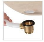
Ensuring the rubber washer is correctly aligned, pass the bath waste clicker through the bath and secure to the waste body assembly.
