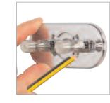
Prepare pipe work from the processor to the required position for the wall spout outlet using Ø15mm pipe. Trim the pipe to a length of 50-60mm measured from the wall surface using a rotary type cutter. If a hacksaw is used the pipe end must be carefully de-burred and chamfered.
