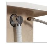
Connect the flexible hose to the blended supply pipe ensuring a suitable non restrictive double check valve is fitted in line with current Water Supply Regulations (not supplied).
