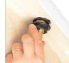
Attach the 15mm push fit flexible hose to the deck spout tail and connect to the blended supply pipe.
