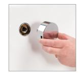
To ensure the spout is correctly positioned at the bottom of the chrome outlet assembly (located on the inside of the bath), it may be necessary to first remove the waste pipe from the outlet body assembly (sited on the back of the bath). Place the chrome outlet in the correct position inside the bath and secure the body (on the back of the bath) to the chrome outlet, through the bath wall. Reconnect the waste pipe to the body assembly.
