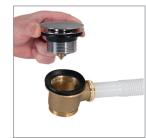
Offer the bath waste into position ensuring the rubber washer is correctly aligned between the waste assembly and the bath base.
