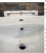
to the protruding bolts and insert the nylon bushings through the wash basin holes (shown below), screw on the flange nuts and tighten using a 15mm spanner. Do not over-tighten.
