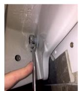
When changing the basin in the future. Just remove the old basin, loosen the screws, adjust the bolts to the corresponding distance of the new basin, re-tighten and re-fit.
