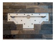
4. Once the plate is in position tile around and up to the edge. The plate can be installed on a pre-tiled surface the wash basin will however stand proud of the wall by 3.8mm but this gap can be filled with silicone.
