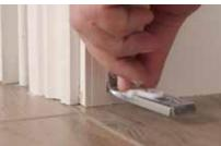
Slot the bottom pivot into the bottom pivot bracket.
