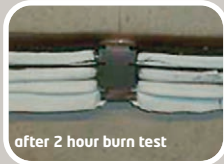
4 new enhanced FP cables
