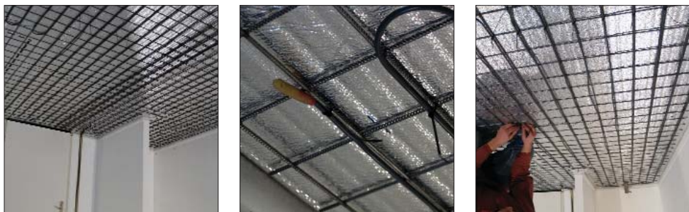
FITTING ON DOVEAILED SHEETING:
