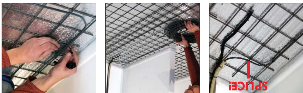
FITTING DIRECTLY ON TOP OF INSULATION:
