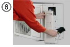
Remove cover of the Quick-Connection
