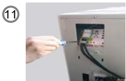
Install fixing clamp
