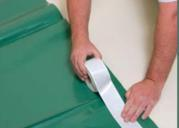
Apply Radbar Double Sided Tape to the membrane, 50mm from the edge. It is very important that the membrane is dry and free from dust and dirt.
