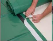
The second membrane must be unrolled overlapping the first membrane by 150mm. Remove the protective paper from the Radbar Double Sided Tape; apply pressure to the membrane while joining the two membranes together.
