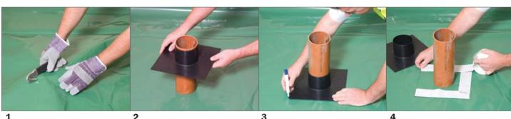
Cut a hole in the membrane to expose the pipe, ensure the hole fits the pipe as close as possible.
