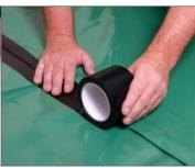
Seal the two membranes by installing Radbar Single Sided Tape to the edge. (ensure that the membrane is completely dry, free from dust and dirt.
