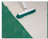
Unroll the first membrane, ensure the surface is dry and free from dust or grease. Inspect the membrane to ensure that there are no indentations or protrusions. If there are remove and apply sand blinding.
