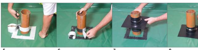
Below the point marked on the pipe. Apply one length of the tape around the pipe.
