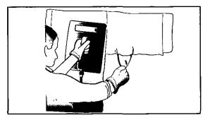
Move the steam plate to the section immediately next to where you have just been working and use a wallpaper scraper to remove the section that has just been steamed. By working in this way you should be able to remove paper continually. You may have to leave the plate against the wall for longer periods with some papers or re-steam if not completely removed.
